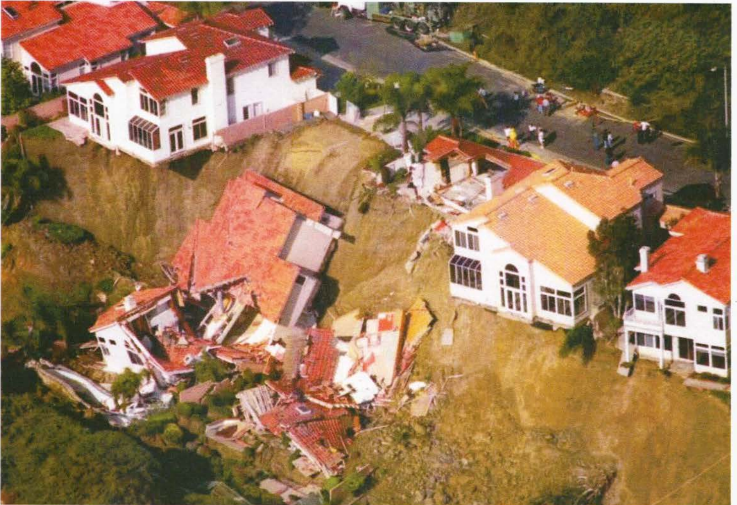
Aerial view of two homes on Via Estoril in Laguna Niguel that fell in 1998 when a rain-soaked hillside collapsed. (Geraldine Wilkins-Kasinga / Los Angeles Times)
